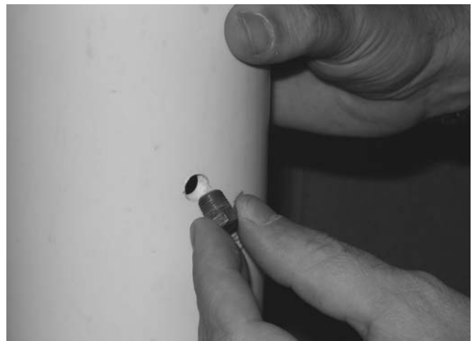
Figure 9.3: Insert Pipe Plug into Test Port
