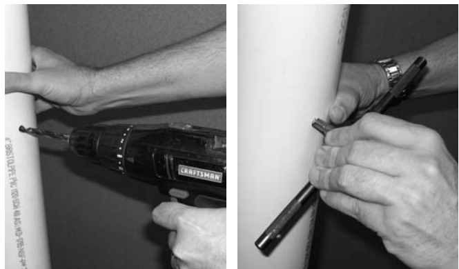
Figure 9.1: Drill and Tap Combustion Test Port
